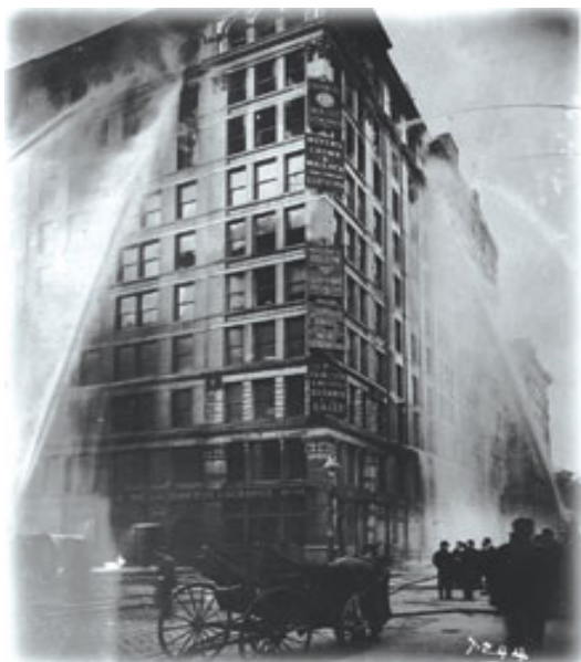
The Asch Building on fire
